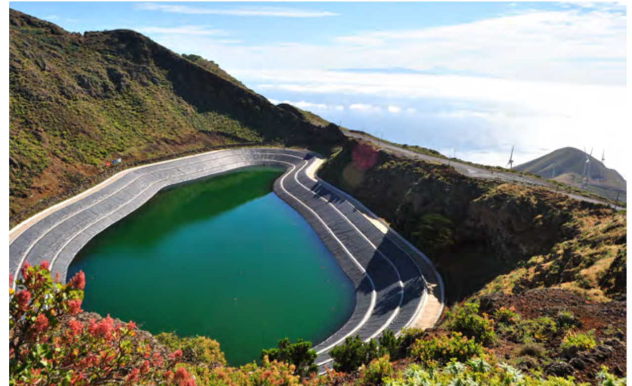
↑ Pumped hydro picture from El Hierro which has received support of the capital investment by the Spanish Government and EU grant through 5 th Framework Programme. The island has received a second prize for Responsible island from EU. © Gorona del Viento.
