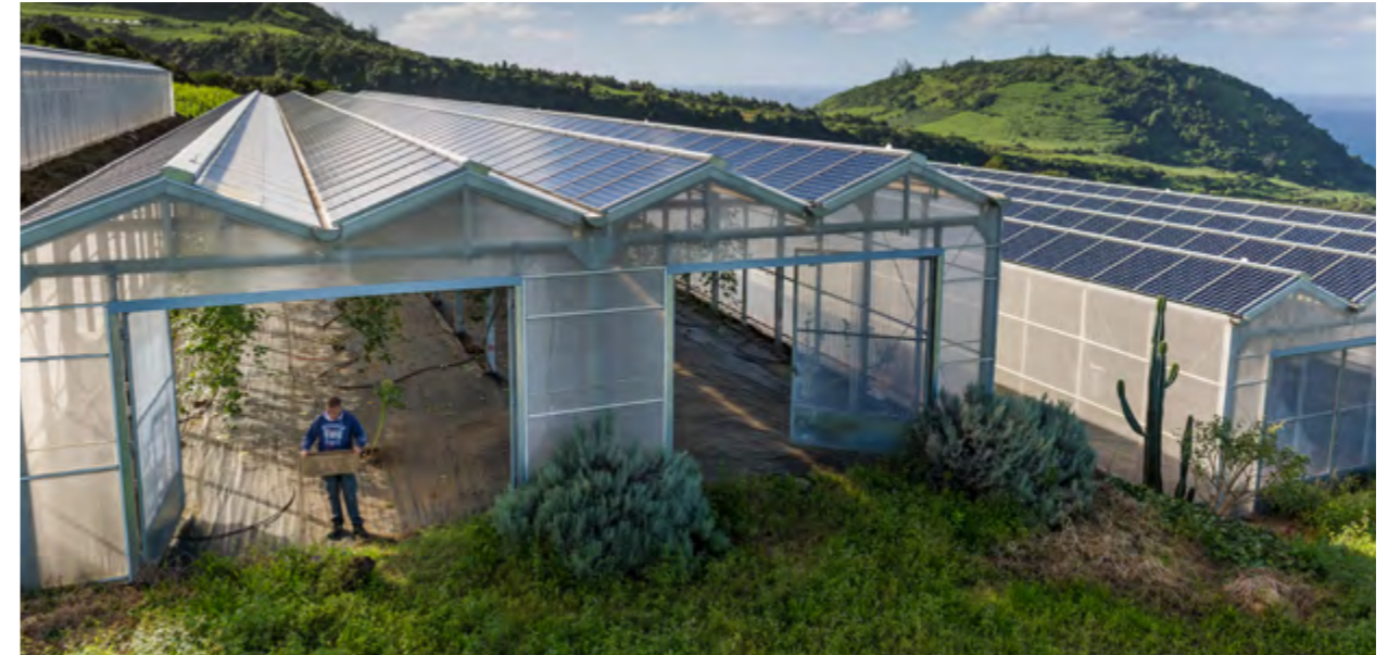
↑ La Réunion has shown how synergies between renewable energy and agriculture can happen thanks to a project of PV integrated into greenhouses. Five of such greenhouses have already been developed on the island. © Photo Akuo Agri.
