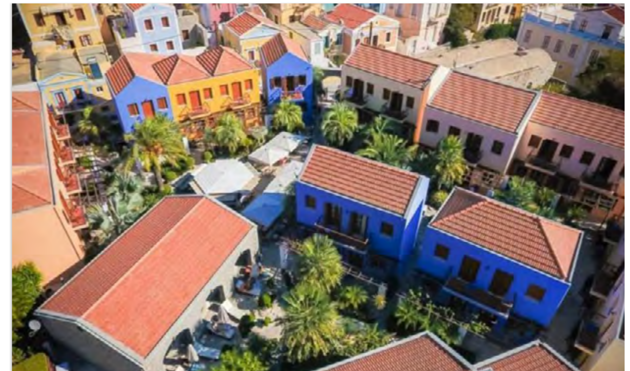
↑ Iapetos Village Hotel in Syros covers 95% of its hot water needs through solar collectors, resulting in savings of 7,440 kg CO 2 annually. Payback time of the investment was 4.5 years, proving that solar thermal technology is a cost-efficient and environmentally friendly way for hot water production. © Photo Nikolaos Mavrikakis.
